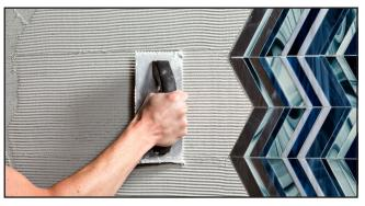
**Step 2** To establish the proper depth of the setting bed, use a  $3/16" \times 1/4"$  v-notch trowel to apply additional thinset and comb full notches in one direction.
