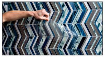
**Step 5** After a full 24 hours (some installations may require extended cure times) starting at the corner; peel the plastic from the tile.
