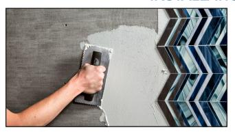
**Step 1** To initiate the bond coat, use the flat side of a trowel and firmly apply thin-set to the substrate.
