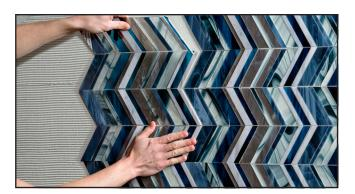
**Step 3** Apply mosaic sheets to the thin-set setting bed, plastic film side out, with light, even pressure. Periodically, check thin-set for skinning (slight drying). If skinning occurs, remove thin-set and reapply.
