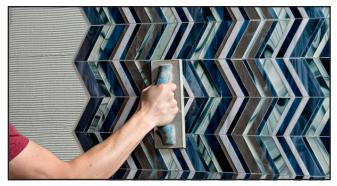
**Step 4** To achieve the flattest possible surface, lightly tap the sheets with a rubber grout float. Pay particular attention to the sheet-to-sheet intersections.
