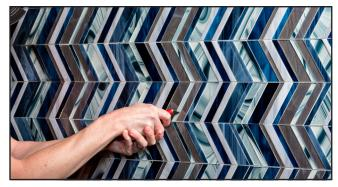
**Step 6** If necessary, remove excess thin-set from the grout joints with a razor knife prior to grouting.
